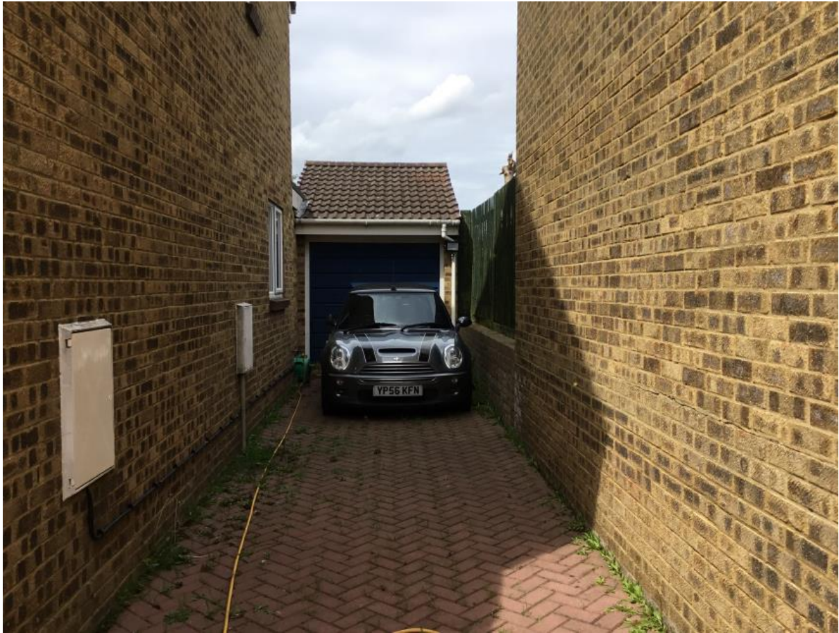
Existing driveway and garage. Side wall of no.22 Harrier Drive.
